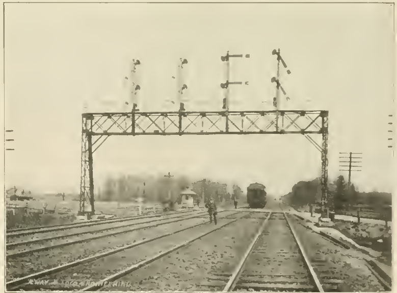
TYPICAL SIGNAL BRIDGE, BLOCK SYSTEM.
